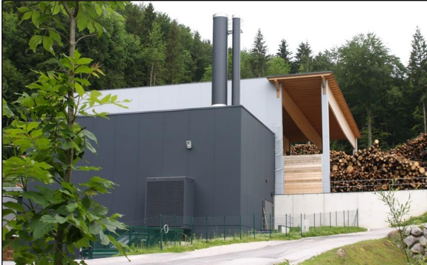
Heating plant in Fuschl am See.
