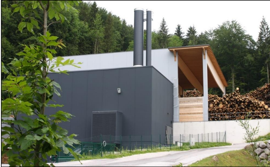
Heating plant in Fuschl am See.
