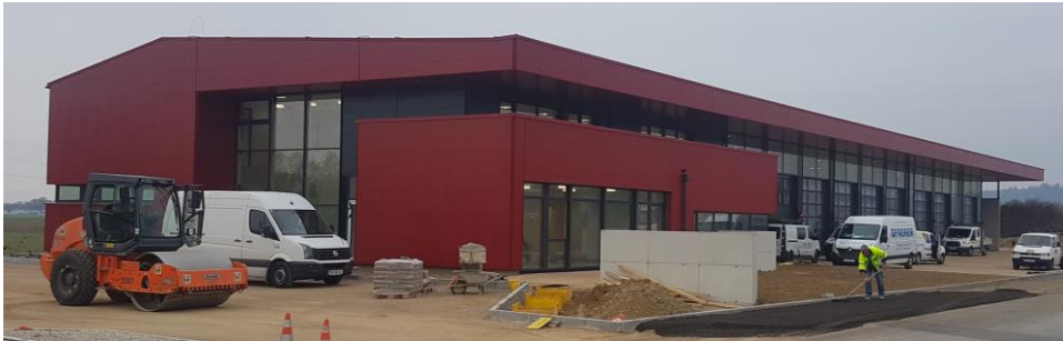
new firefighting department
