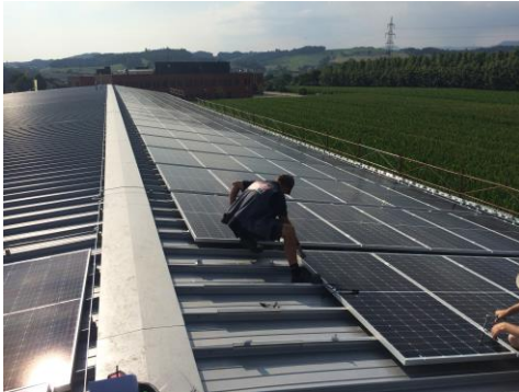
installation of PV
