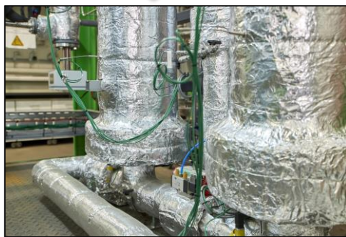
Gas cleaning on our gas-cleaning test-rig.
